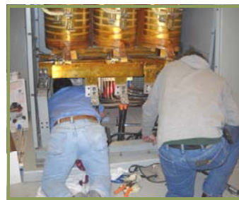
Tightening of transformer buss duct
